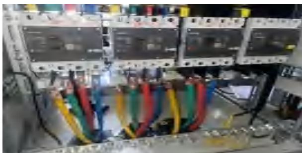
箱变低压侧电缆缺失标牌
